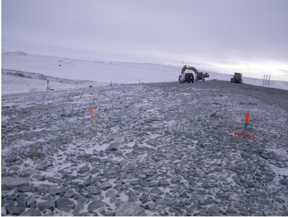
Photo 6: North Dam – Survey stakes marking slightly underbuilt portion of the final ROQ crest on the upstream side.
