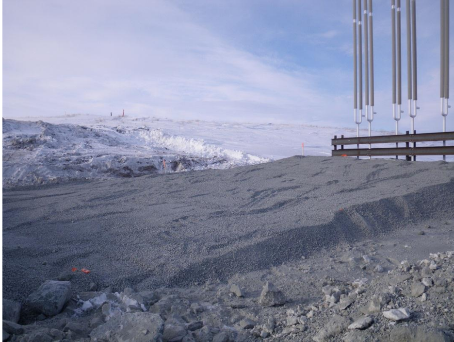
Photo 4: North Dam – View of crush placed over thermosyphons pipes; this material still requires compaction.
