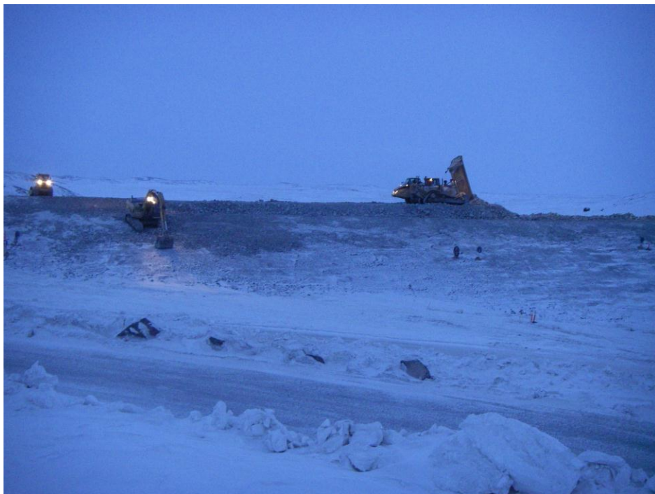
Photo 9: North Dam – progress photo of dam construction. Excavator finishing the downstream slope and truck dumping ROQ at the placement front. Photo looking west from Tail Lake Road.
