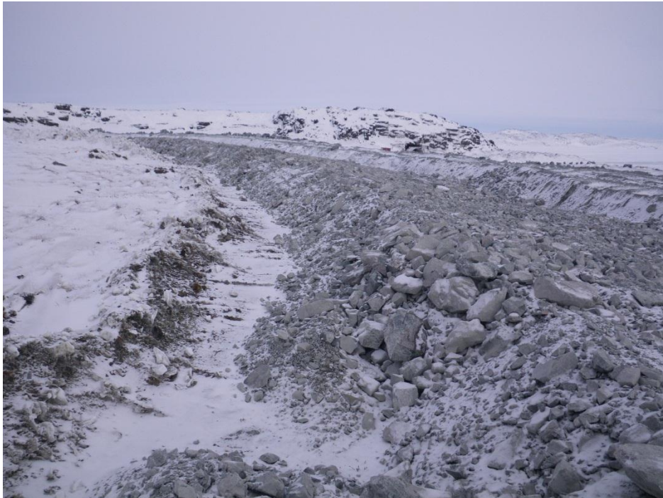
Photo 7: Diversion Berm – culverts after backfilling with second lift of ROQ material.
