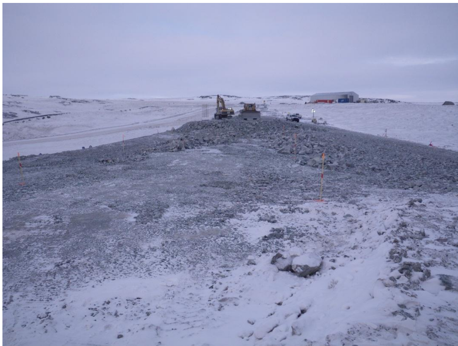
Photo 5: North Dam – View of remaining ROQ to be placed at the end of dayshift. Looking north east along the dam alignment from approximately station 1+20.
