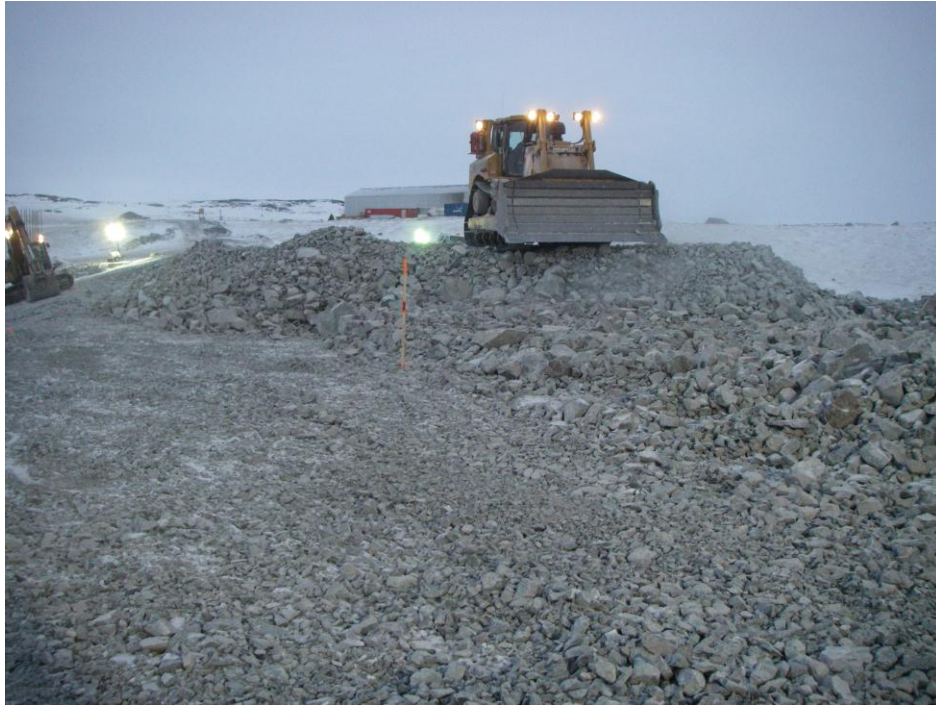
Photo 8: North Dam – dozer placing ROQ on the final lift. Photo looking north-east from station 0+40.
